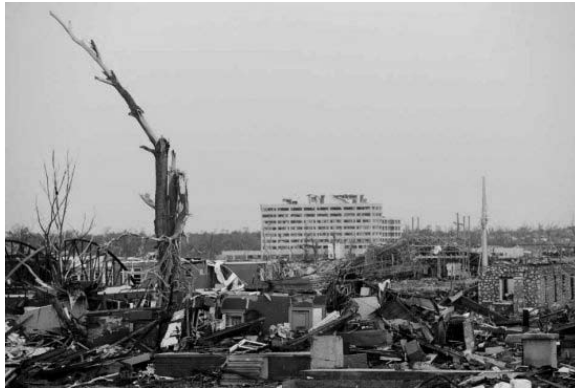
The hospital in the background of what is left of homes after a large tornado hit the town of Joplin, Missouri, USA, 23 May 2011. The tornado caused damage to a large portion of the town and the city's hospital and school. Photo: EPA/Larry W. Smith
